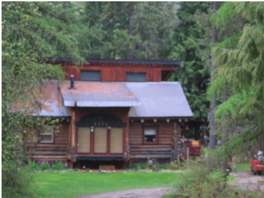
Figure 2. Photograph showing wooden siding and litterfall present on some homes within the wildland urban interface.
